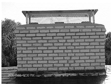
Metal Cap on Clay Liner Chimney Top
