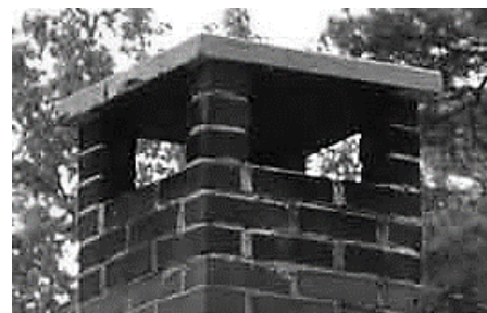
Concrete Cap Chimney Top
