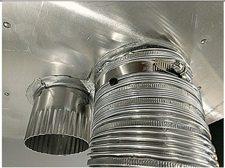
Hose Clamp first. Secure w/ Screw above Hose Clamp
