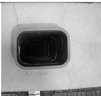
Clay Tile Liner Flue
