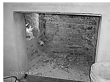
Badly Deteriorated Firebox
